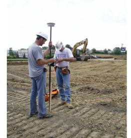
Construction Layout with Robotics and GPS
